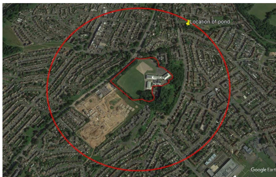
Figure 3 – Red circle indicates a 500m buffer around the proposed development site. The yellow pin indicates the location of the pond located within 500m of the proposed development site. Image used under licence (©2022 Google). Imagery date 20/07/2021.
