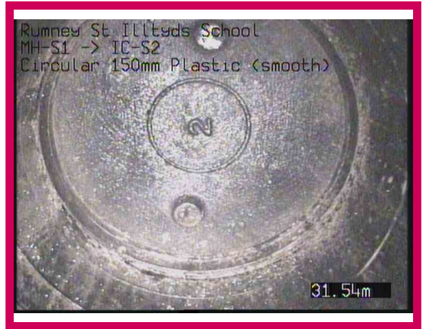
2, 00:05:41, 31.54 m Finish node, inspection chamber, reference: IC-S2
