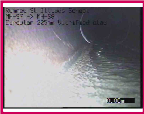
1, 00:00:00, 0.00 m Start node, manhole, reference: MH-S7
