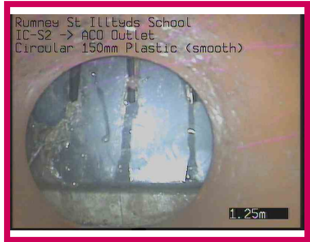
2, 00:00:31, 1.25 m Finish node, other special chamber, reference: ACO Outlet, Aco channel basket outlet
