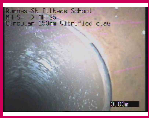
1, 00:00:00, 0.00 m Start node, manhole, reference: MH-S4
