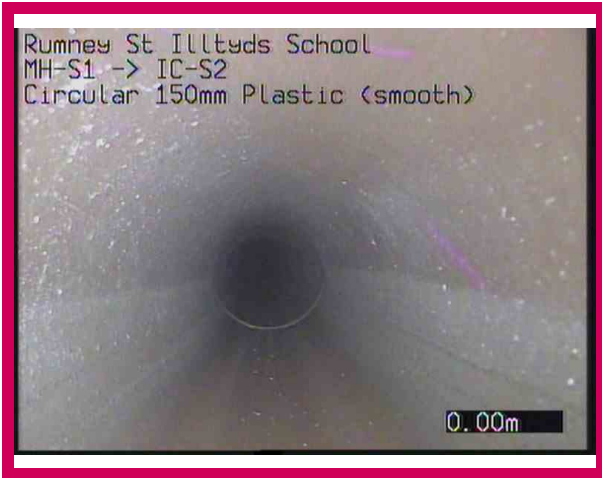
1, 00:00:00, 0.00 m Start node, manhole, reference: MH-S1
