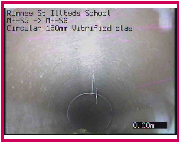
1, 00:00:00, 0.00 m Start node, manhole, reference: MH-S5
