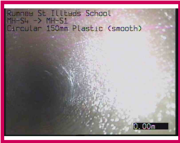
1, 00:00:00, 0.00 m Start node, manhole, reference: MH-S4
