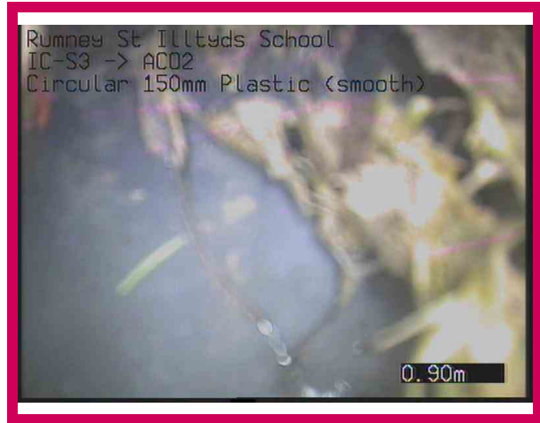
2, 00:00:30, 0.90 m Finish node, other special chamber, reference: ACO2, Aco channel basket outlet
